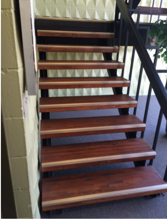
Stair Tread Replacement
